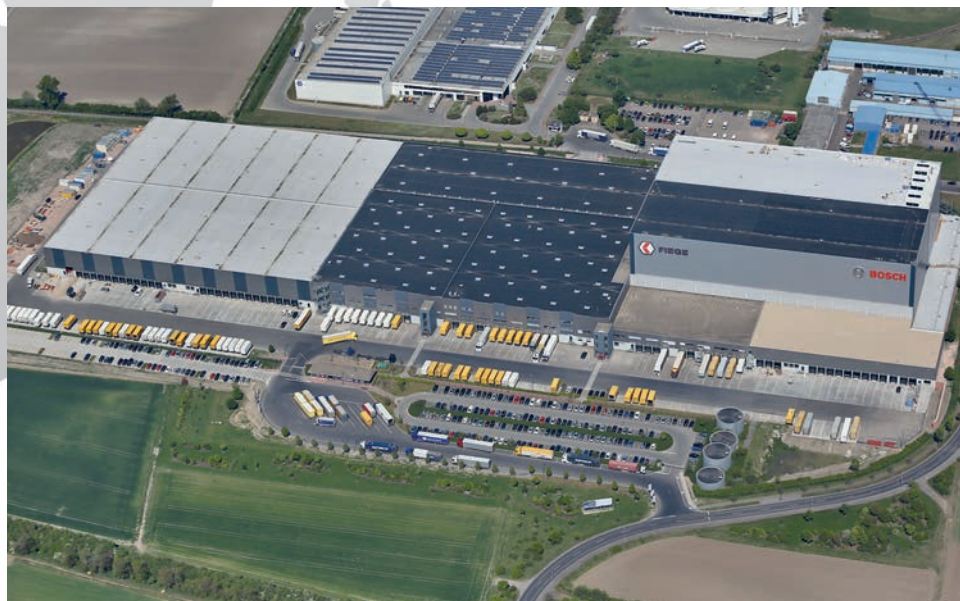
To the left of the picture, the structural expansion is visible, as are the light rooftops to the right.
