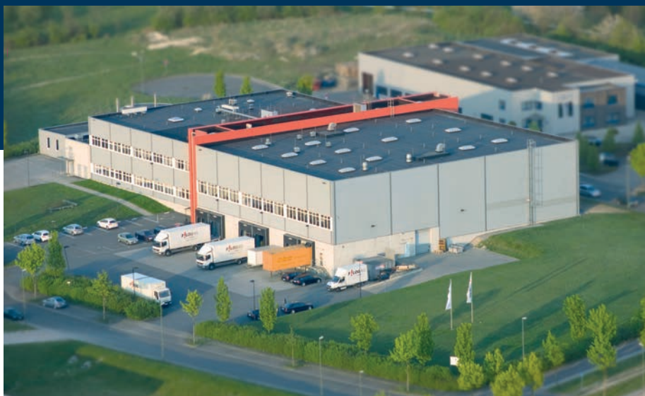
The Medical Order Center in Ahlen supplies a broad product range to around 50 hospitals
