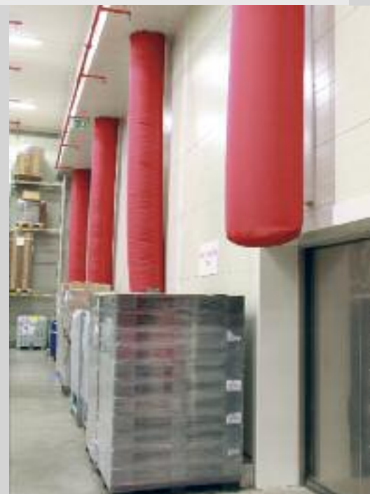
The red hoses inside the cold houses secure a steady flow of turbulence-free cold air.
