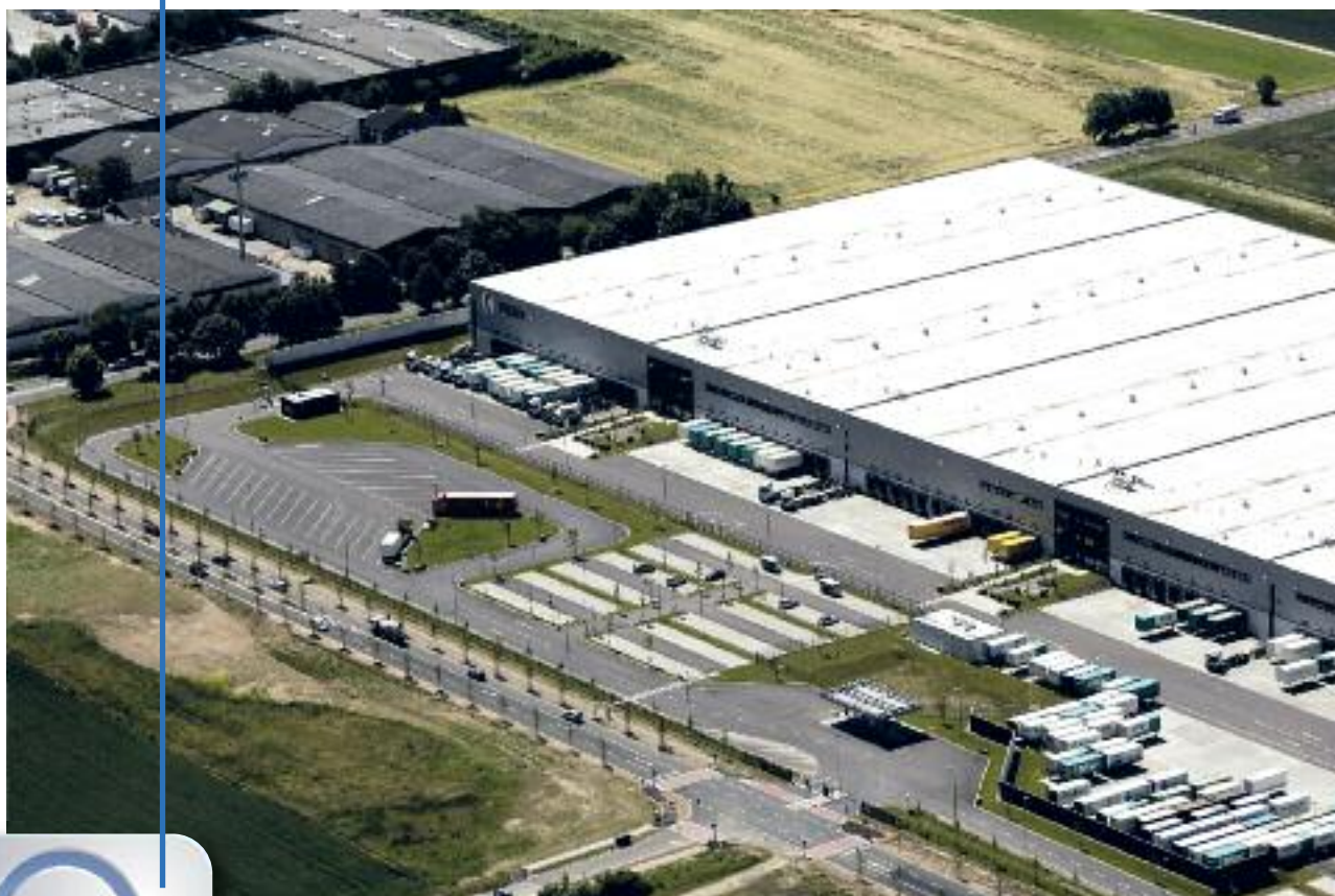
Access control and video surveillance at large facilities like Neuss are elements of Security Management standards.
